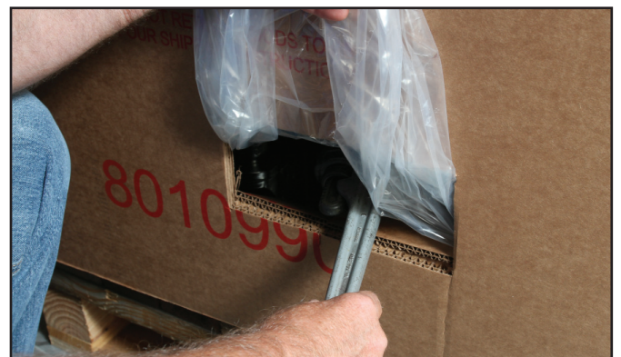
Figure 3: Cut a 9"x5" hole centered on the marked spot with its top edge 10" above the box base, which will provide access to cap the gas manifold.
